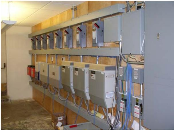
Fig. 1: Inverters at the AEC PV Test Facility. Two SMA 2500s, one Fronius 2500, two SunVista 3500s, and three PV Powered 2800s.
