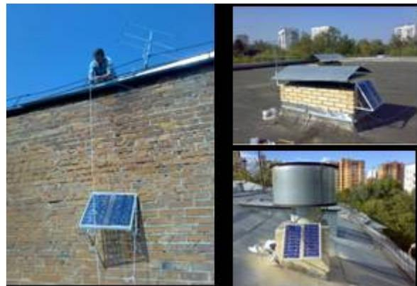
Fig. 3: Installing of aerial and solar module on the roof of school №1533 (left) and solar module on the roof of schools №390 (top right) and №1277 (below right)
