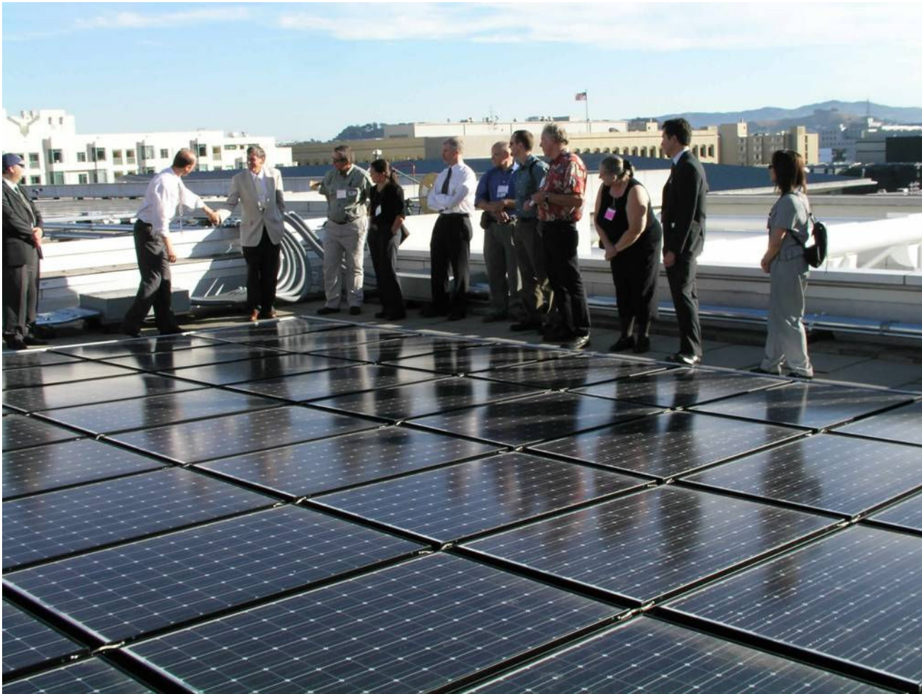
Dan Shugar of Power Light greets Frank Vignola and participants of the Solar Cities Summit before giving a close up view of the 675-kilowatt solar array atop the Moscone Center. The system supplies as much as 1/3 of the center's midday electricity demand. Photo by Ben Chan
