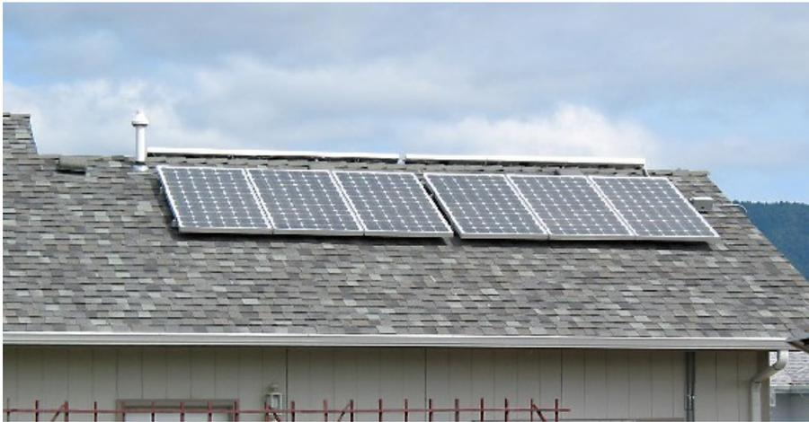
*West facing array installed on the roof of Bob Maynard's garage. The top of the east facing array can be seen along the roof line. The south facing array is not shown in this picture. Since each array group receives peak power at different times, the inverter needs to handle three different strings.*
