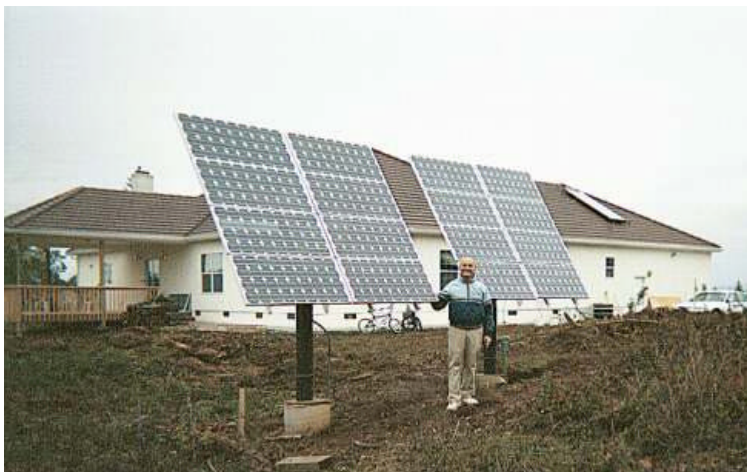
Ground mounted PV panels for Solar electric home. Photo courtesy Energy Service Company.
