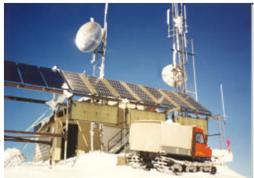
The state of Idaho uses PVs to power communication systems. This installation is at Pilots Peak. (Photo courtesy of the Department of Administration)
