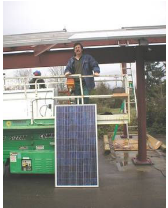
Equipment is needed to help lift 144 panels.
