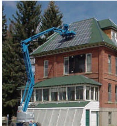
*A crew from Solar Plexus installs PV array for NCAT (NCAT photo)*
